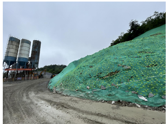
搅拌站砂石料临时苫盖
