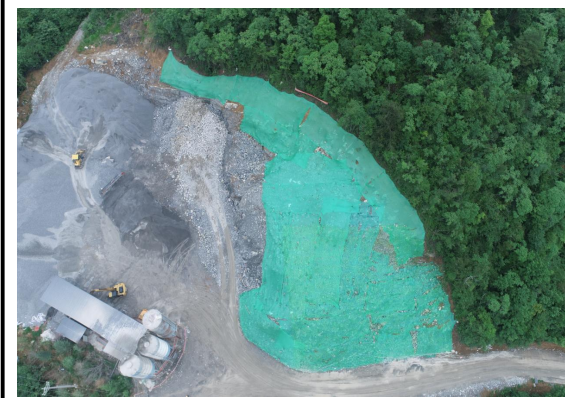
搅拌站砂石料临时苫盖
