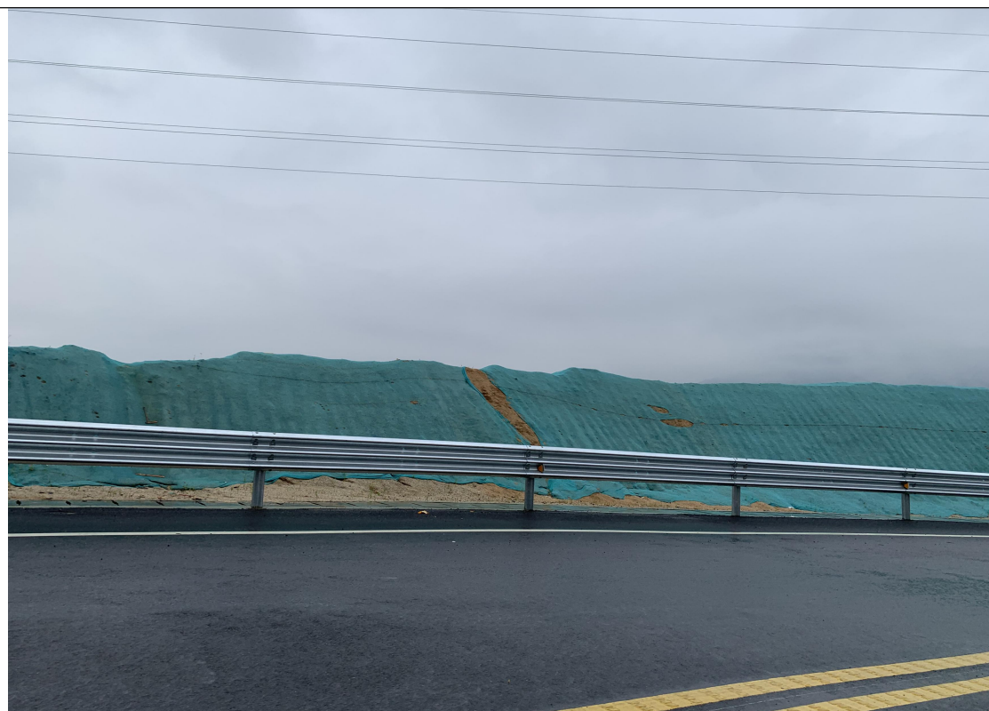
边坡临时苫盖
